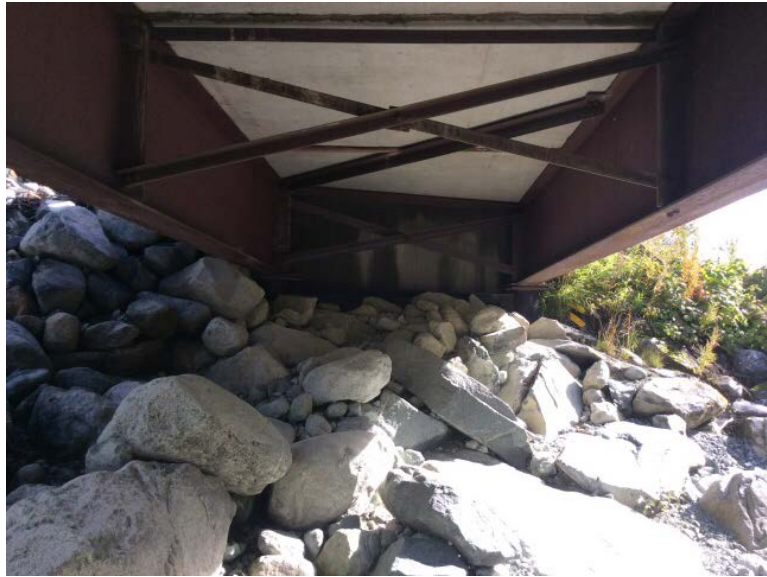
Left Bank Abutment when facing downstream
