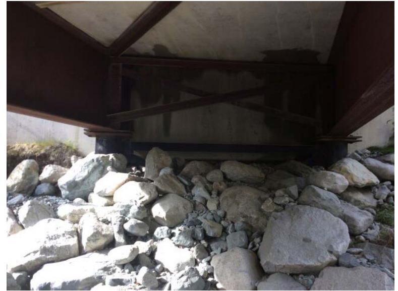
Right Bank Abutment when facing downstream
