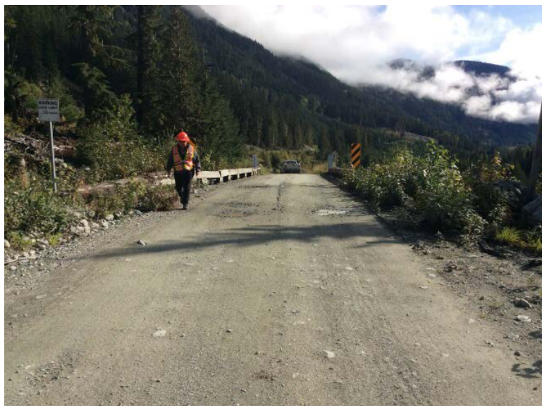
Approach from Right Bank when facing downstream
